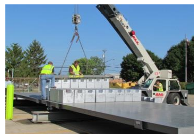
90% of the concentrated load capacity (CLC) is loaded onto the weighbridge twice
